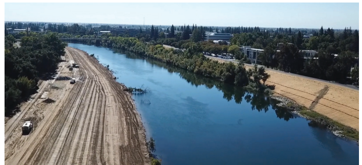
Bank protection work conducted by the US Army Corps of Engineers.
