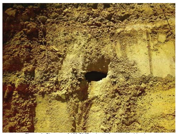
Figure 4. Closeup of 18" CMP culvert along waterside slope
